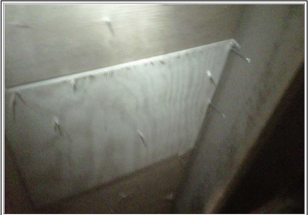
Patched sheathing in attic areas.
